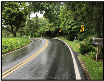
Center lines and edge lines are common pavement markings on a road.
