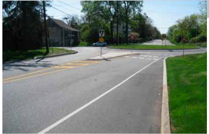
Under the state Greener and Safer Intersections Act of 2012, Pennsylvania has invested $35 million around the commonwealth in replacing traditional signalized intersections with modern roundabouts.
