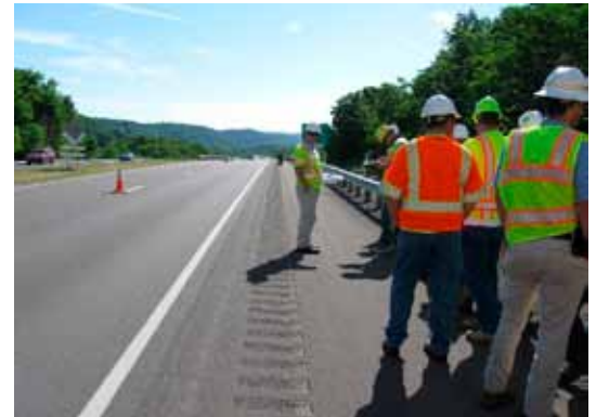
This 6.3-mm thin asphalt overlay is applied on SR 220 in Lycoming County. The specification for this pavement preservation technique was recently approved for incorporation into PennDOT Publication 408 and will take effect April 2018.
