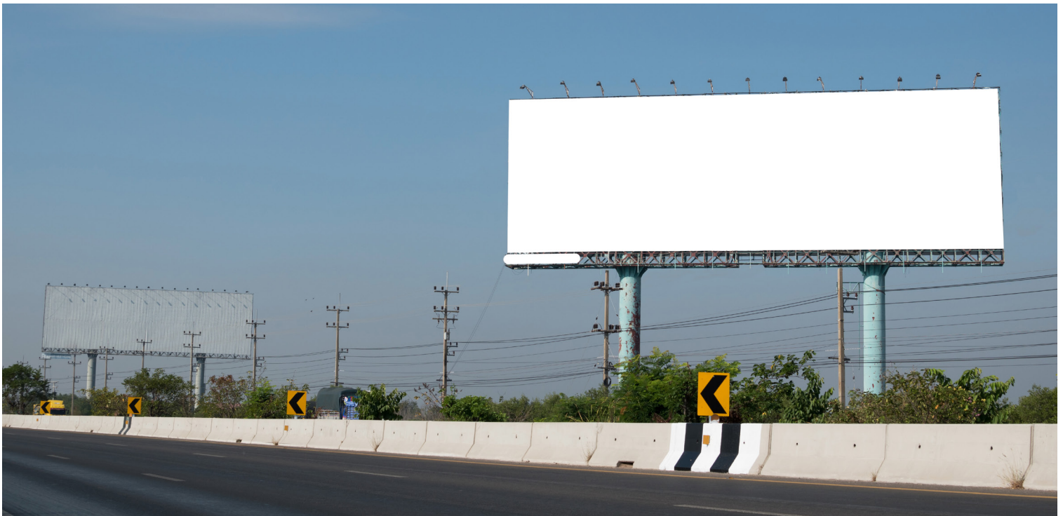
Under federal law, PennDOT must effectively control outdoor advertising within 660 feet of an interstate or primary route.
