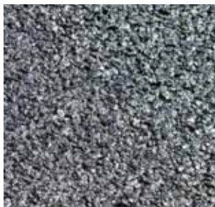
UTWC seals the pavement, reducing oxidation and weathering of the surface. It has a service life of 8 to 10 years. (PennDOT photo)
