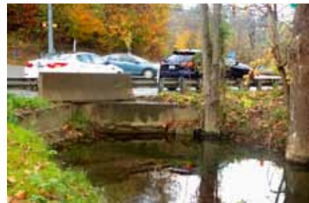
At an intersection of a state and township road in Allegheny County, PennDOT is planning to relocate a small bridge while improving an enclosed surface water drainage facility and headwalls. Photo by Harry Funk, The Almanac .
