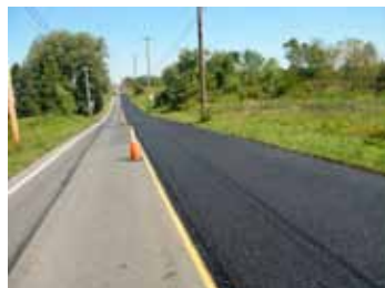
UTWC can be constructed one lane at a time without matching lanes before opening to traffic. Construction requires only a short, single-lane, moving traffic closure. (PennDOT photo)
