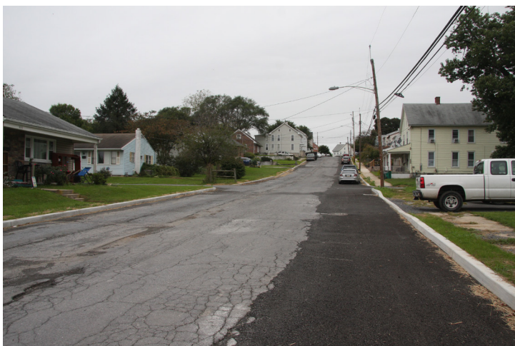
Planning for a full-depth reclamation project begins about two years earlier when the borough makes improvements to utilities and curbing on the targeted road.
