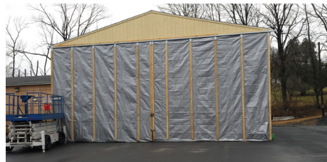
2017 Winner: Salt shed entrance curtain, Whitehall Township, Lehigh County
