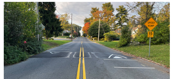
Speed cushions implemented in Susquehanna Township, Dauphin County can slow traffic on a more suburban section of road. Photo: PennDOT LTAP
