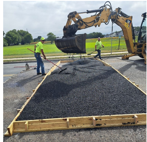
The township filled the speed table form with asphalt.
