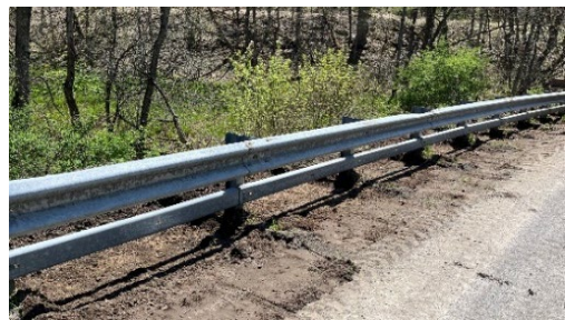
The guide rail after being cleaned.
