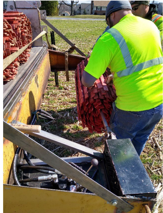
Penn Township came up with a way to use the hydraulics on its small dump truck to create a winder that rolls up the fencing on a metal rod. The new equipment has increased the efficiency of rolling the snow fence into tighter rolls for storage. Photo: Penn Township, Lancaster County
