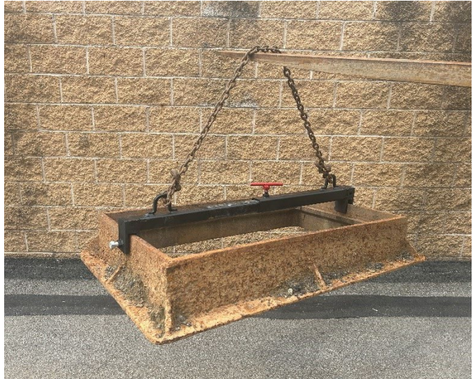
Peters Township designed a tool to safely and conveniently lift storm basins for maintenance.
