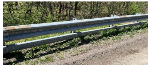
The guide rail before cleaning.
