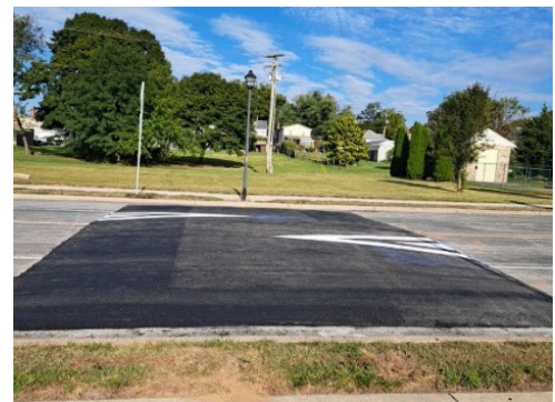
The township added the sides and markings on the speed table. Photos: South Londonderry, Lebanon County
