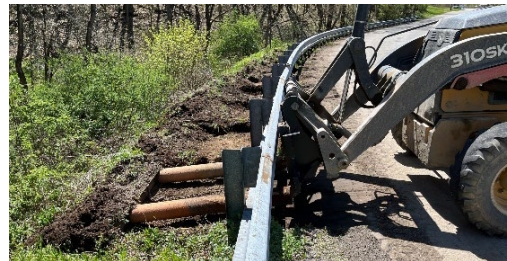
The guide rail being cleaned.
