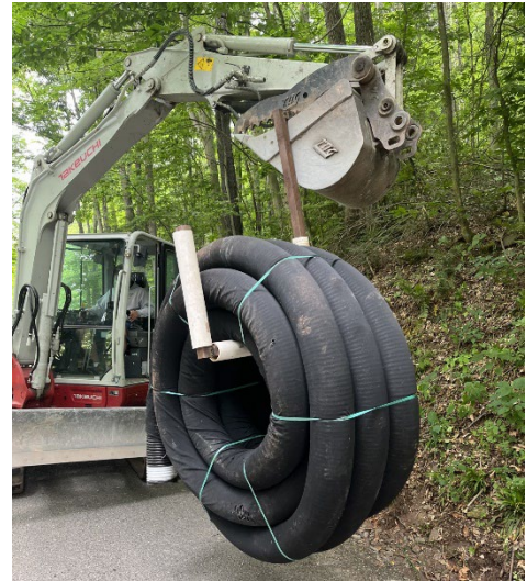
The Un-Reeler assists with the transport and installation of both 100 feet long reels of 6 inch diameter underdrain and 60 feet long reels of 8 inch diameter underdrain. Photo: Lewis Township, Lycoming County
