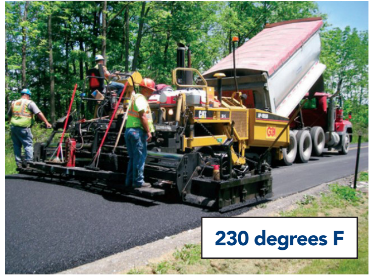
The lower fumes associated with warm mix asphalt result in a safer work environment.
