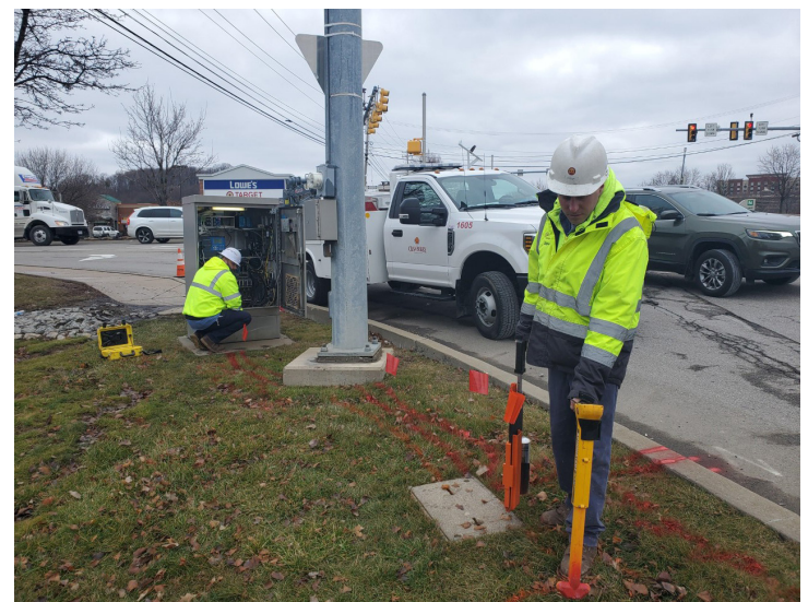
Municipalities that own facilities must be members of PA One Call and mark their utilities upon notice that digging is to occur.
