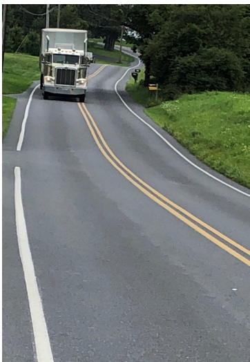
Act 31 of 2018 allows larger trucks to access certain state and local roads that were not previously open to truck traffic.
