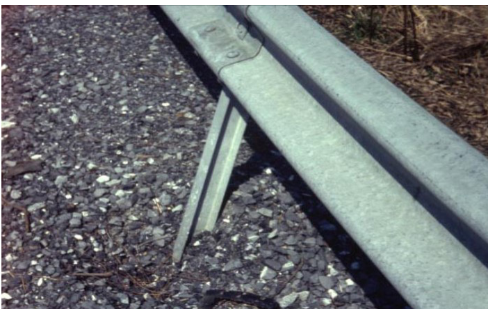
Low-severity post deflection
