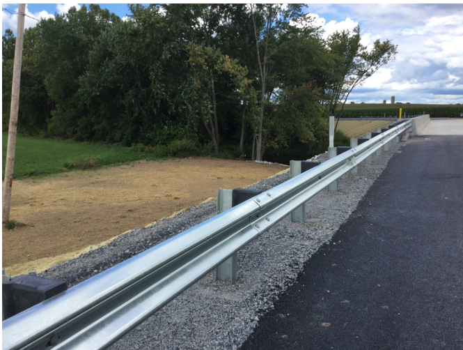
A guide rail helps to shield vehicles that run off the road from hitting natural or manmade obstructions.
