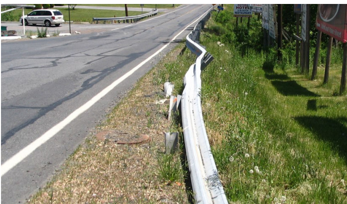
Damaged turned-down end treatment and W-beam guide rail
