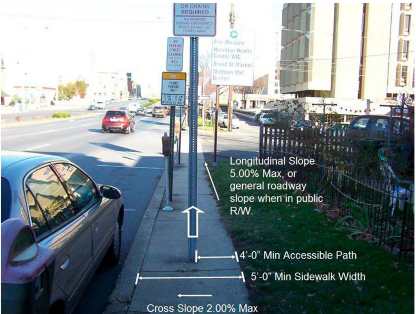
A pedestrian-accessible route has certain requirements.
