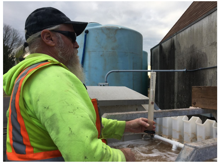
A worker uses a salometer to test for the proper brine mixture. A glass sodium chloride hydrometer costs about $30 and can also be used to measure the percent of saturated salt solution on a scale of 0 to 26.4%. A good rule of thumb to follow while mixing sodium chloride and water is 2.3 pounds of salt per one gallon of water to produce 23.3% brine solution.
