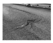
between any of the placed layers of pavement near a turn or stop sign where there is a significant stopping or turning force on the pavement structure.
