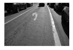
vehicles traveling over the area to continue to compact the area unevenly, or poor subbase/subgrade conditions, which are not able to support the weight of traffic.
