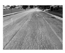
Cracks may be slightly spalled and may be sealed; pumping is not evident.
