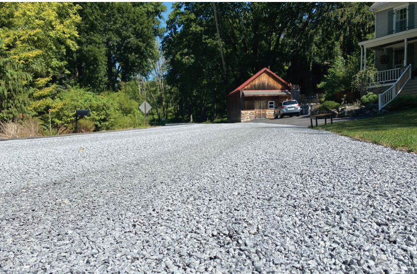
A view of a completed seal coat project along a municipal road in the commonwealth. Photo: PAAMA
