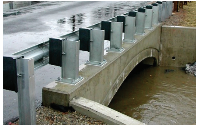
Above, a culvert with an integral top, sides, and bottom and designed structurally to account for soil-structure interaction. Photo: PennDOT LTAP.
