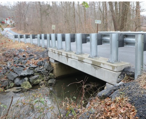
A short-span bridge consisting of reinforced-concrete slab resting on abutments. Photo: PennDOT LTAP.
