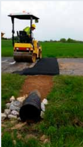
Stormwater pipe replacement project along township road.
