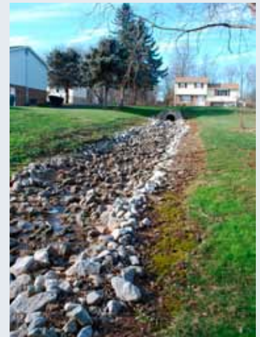
Riprap-lined swale draining toward outfall into a stream.
