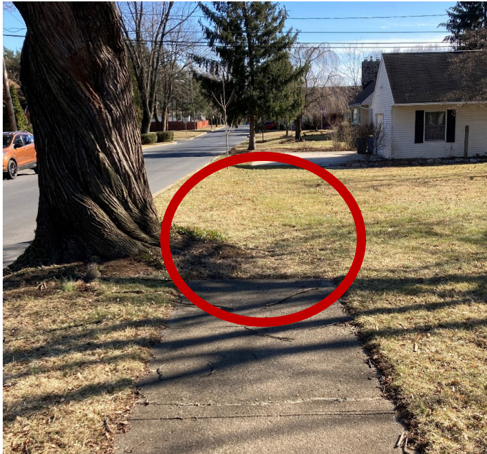
Figure 8: An example of a sidewalk gap in the pedestrian network is shown here. This could lead pedestrians into conflicts with traffic.
