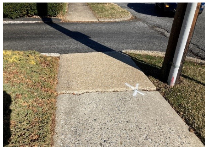
Figure 1: This sidewalk inspection marks the repair location with white marks.
