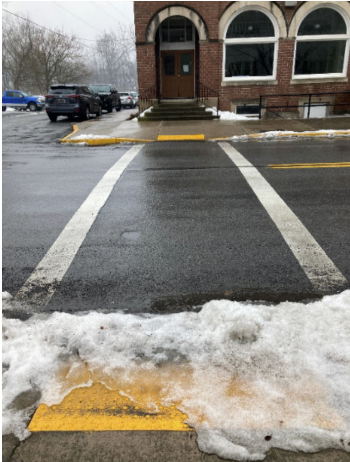
Figure 12: Water, snow, and ice can create barriers to access a sidewalk and/or ramp.
