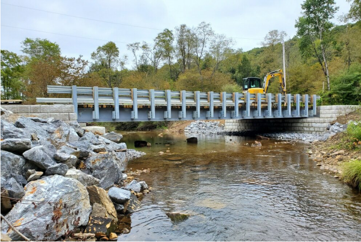
Twin Lakes bridge in Jones Township.
