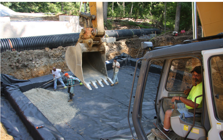
Blymire Hollow bridge under construction in North Hopewell Township.
