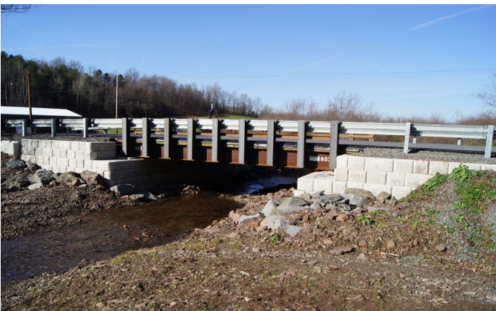
Ensminger Road bridge in Sullivan Township.
