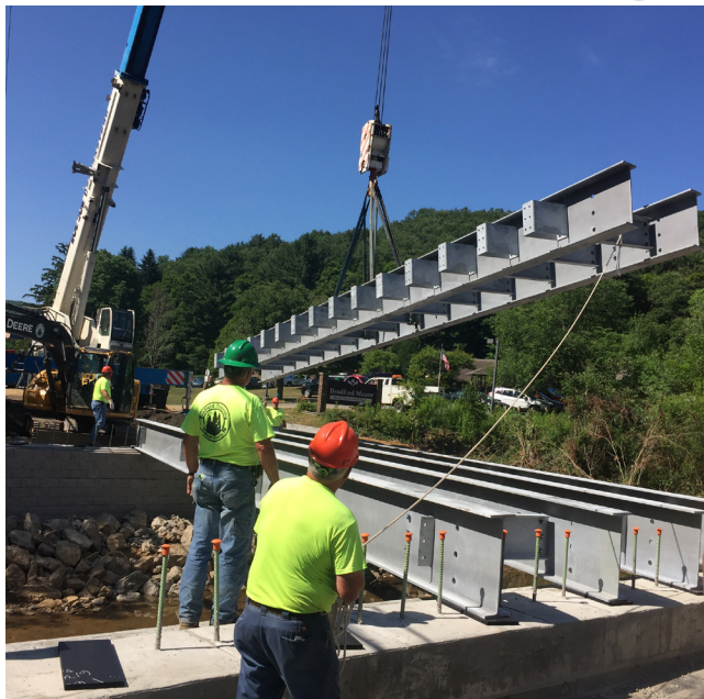
PHOTO OF LANGMAD LANE BRIDGE IN BRADFORD TWP., MCKEAN CO.
