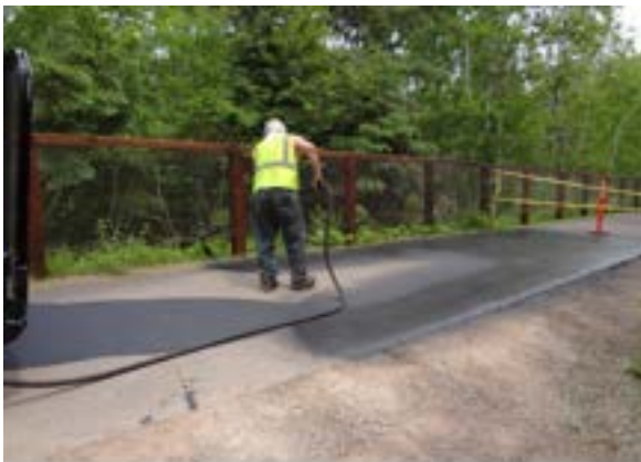
Figure 15-4: Fog Sealing a Shared Use Path
