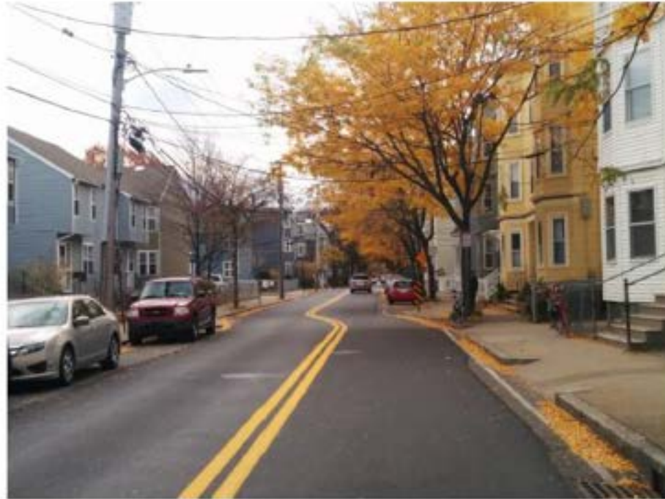
Figure 8-6: Example of a Chicane Treatment Created by Alternating Parking from One Side of the Street to the Other
