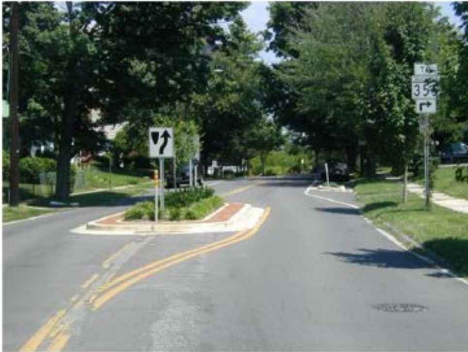
Figure 8-5: Example of a Chicane Treatment on a Two-Way Street Created by a Median and Curb Extensions
