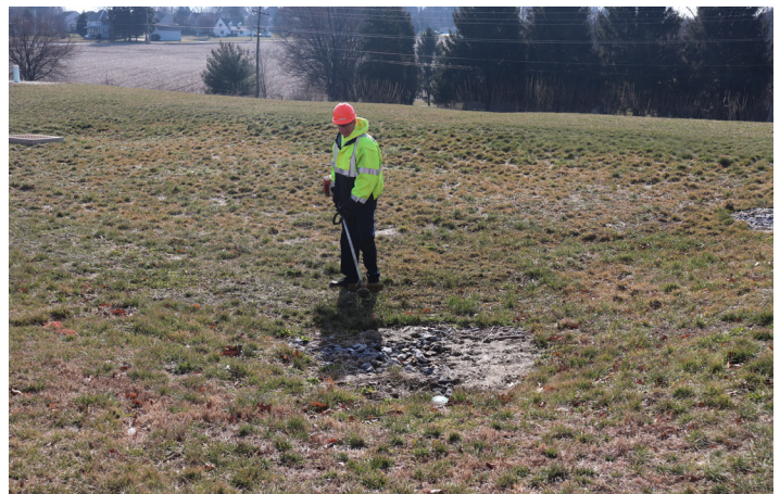
The lightest equipment appropriate for the work should be used on infiltration/ filtration surfaces. Hand-helds like string trimmers are a good choice for vegetation maintenance.
