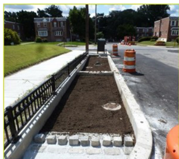
A GSI Street Bumpout to provide traffic calming and stormwater management with uncompacted, engineered soils. Photo: Cedarville Engineering Group
