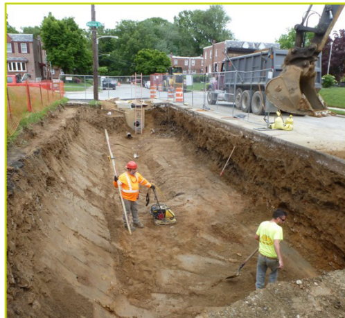
GSI bed bottoms should not be compacted! An exception would be in cases where infiltration is not recommended or possible. Photo: Cedarville Engineering Group
