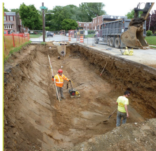
GSI bed bottoms should not be compacted except in cases where infiltration is not recommended or possible. Photo: Cedarville Engineering Group.
