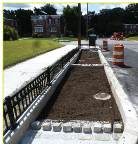
A GSI street bumpout can provide traffic calming and stormwater management with uncompacted, engineered soils. Photo: Cedarville Engineering Group.
