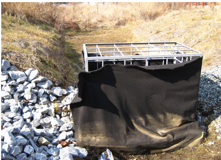
Basin outlet structure with E&S protection during retrofit project.
