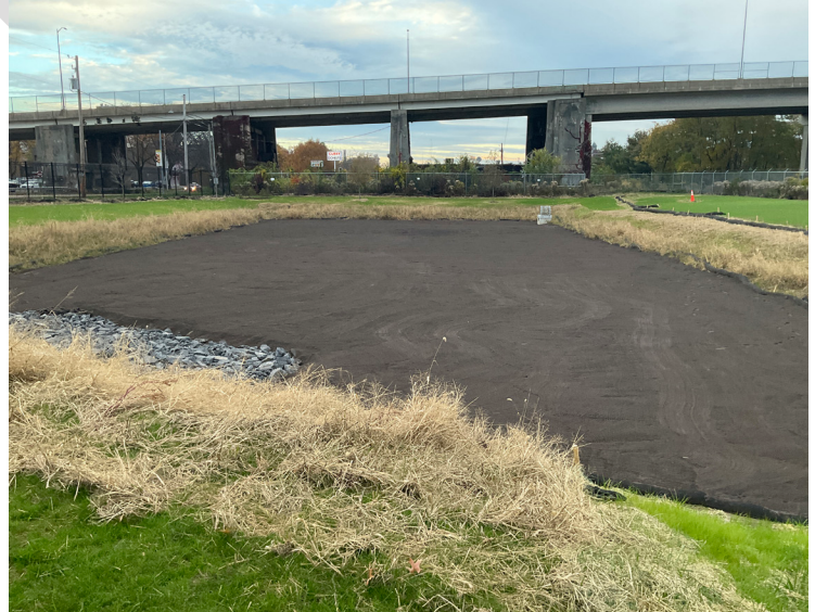
Amended soil placement in basin floor. Photo: NTM Engineering, Inc.
