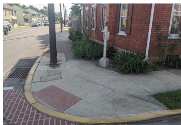
This intersection features signal support with a supplemental accessible pushbutton. Photo: PennDOT LTAP
