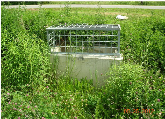
Vegetative overgrowth in a basin can lead to erosion and obstruct flow, both of which can reduce efficiency and overall environmental benefits. Photo: NTM Engineering, Inc.
