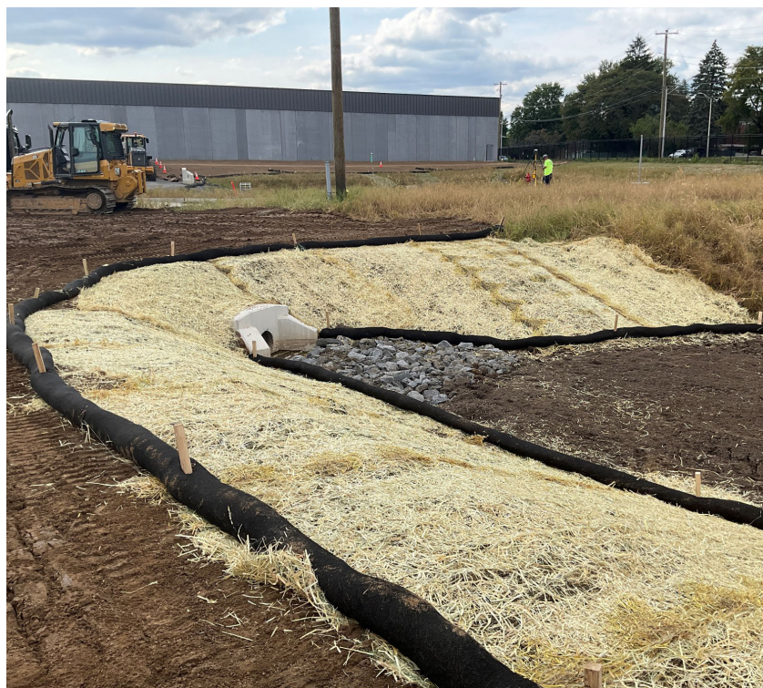
The photo illustrates slope regrading with sediment control measures in place during construction. Photo: NTM Engineering, Inc.
