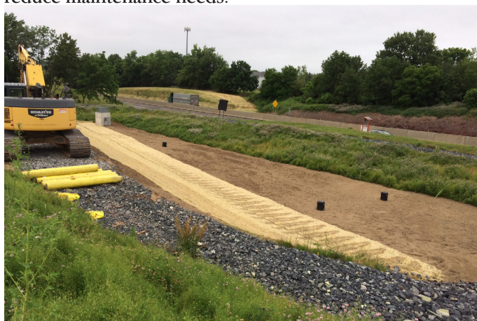
Amended soils in a bioretention facility can improve treatment performance. Photo: NTM Engineering, Inc.
