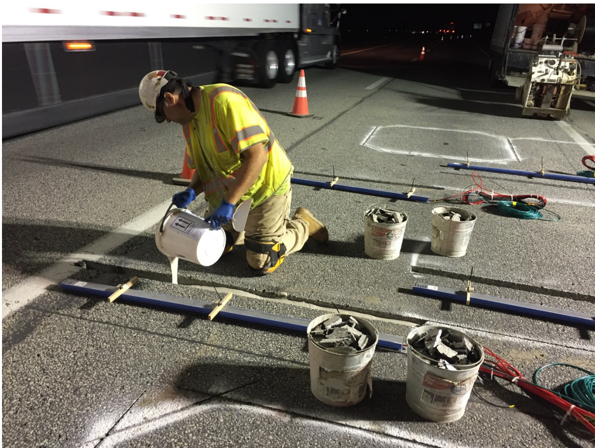
Installation of VWIM 712 in Franklin County
