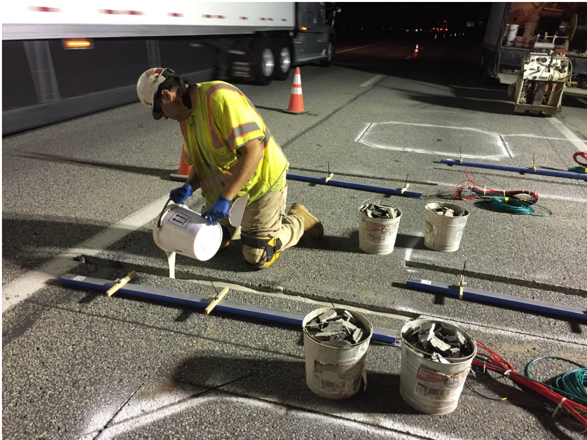
Installation of VWIM 712 in Franklin County
