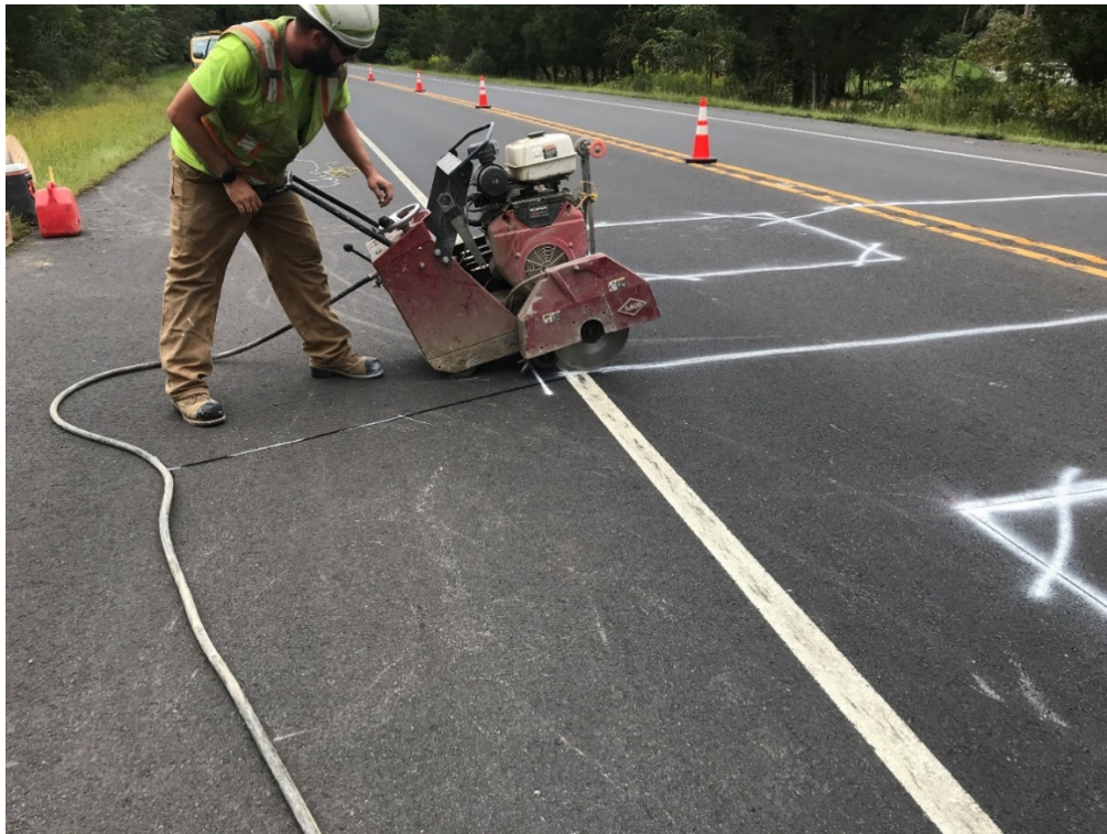
Installation of CAVC 853 in Bucks County
