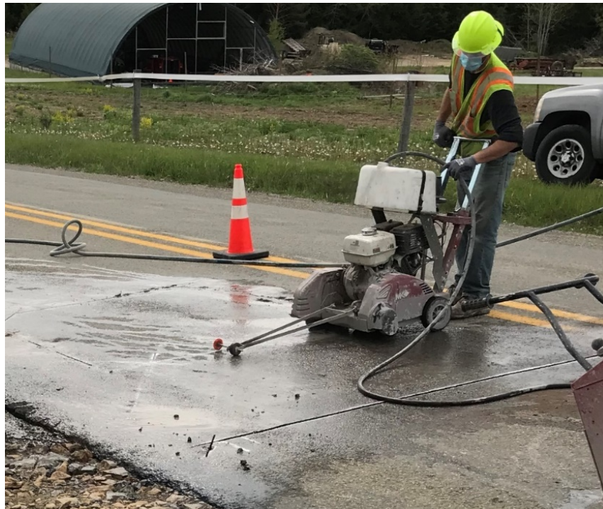
Installation of CAVC 15 in Fulton County
