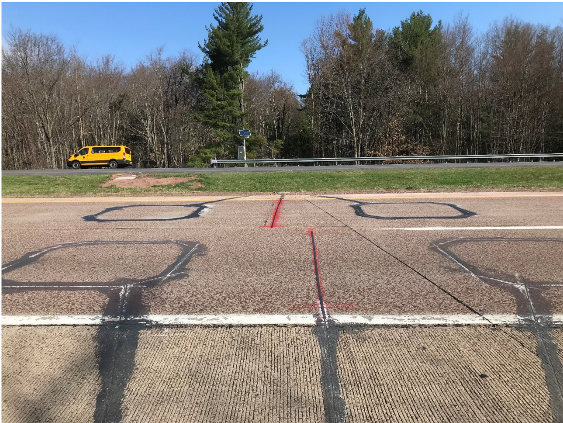
CAVC 392 Sensor Array on I 80 in Luzerne County
