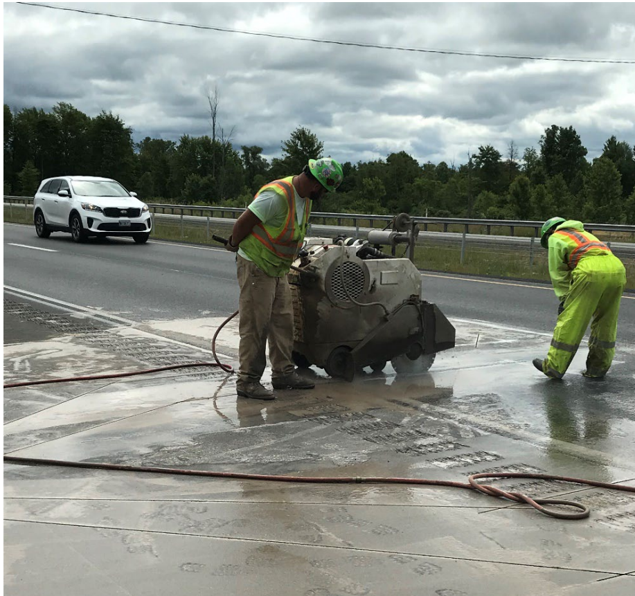
Installation of WIM 713 in Erie County
