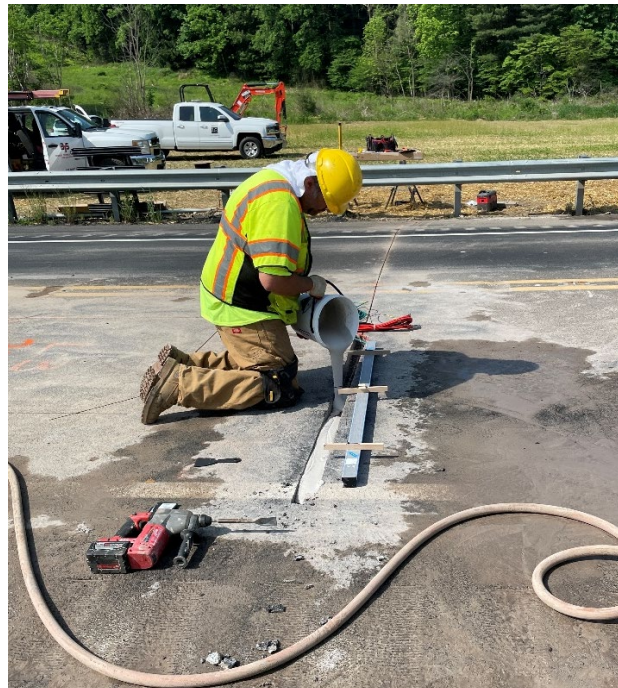
Installation of WIM 700 in Indiana County
