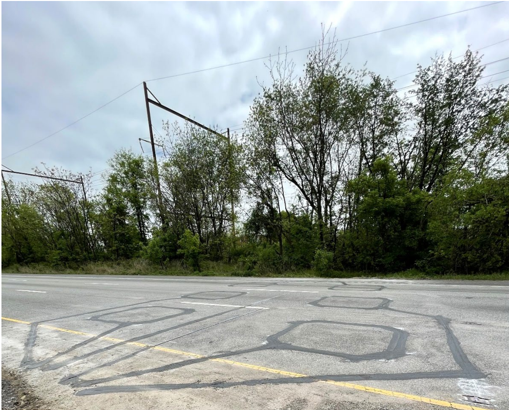
CAVC 13 Sensor Arrays on I 95 in Bucks County
