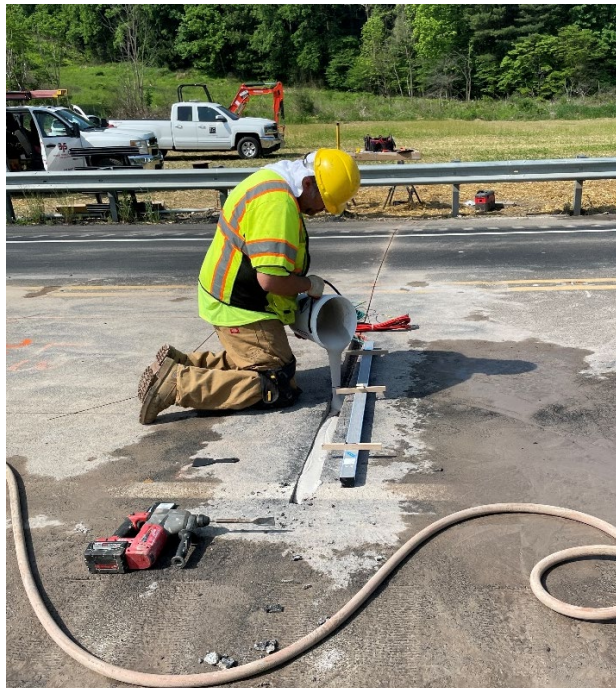
Installation of WIM 700 in Indiana County
