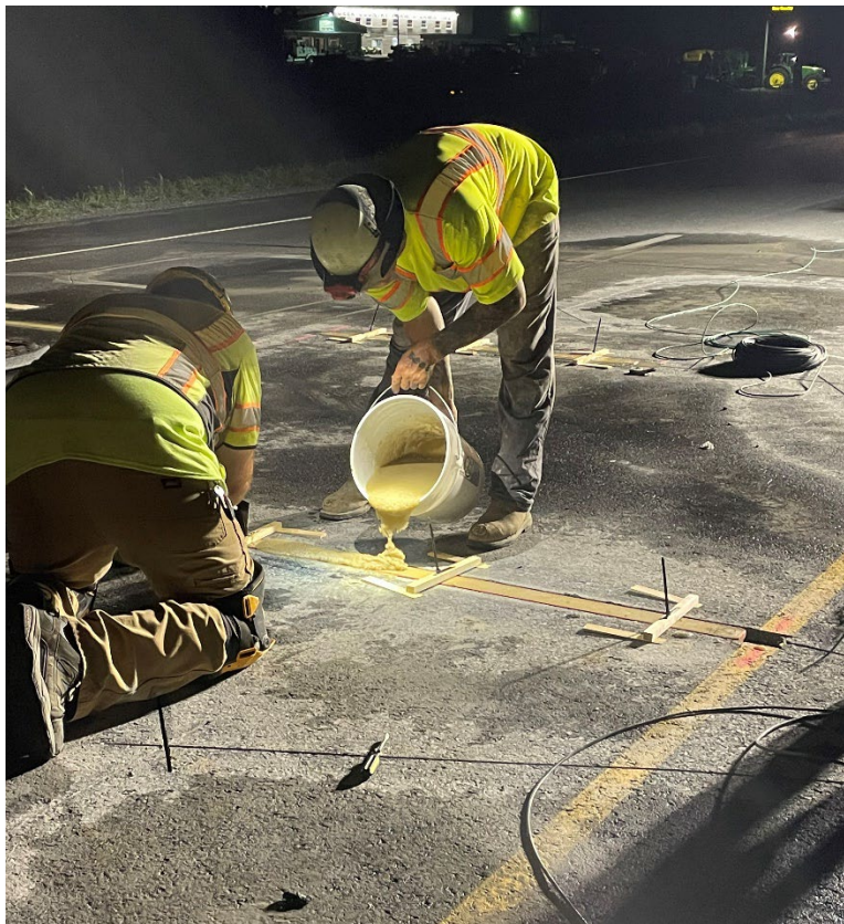
Installation of WIM 703 in Lancaster County
