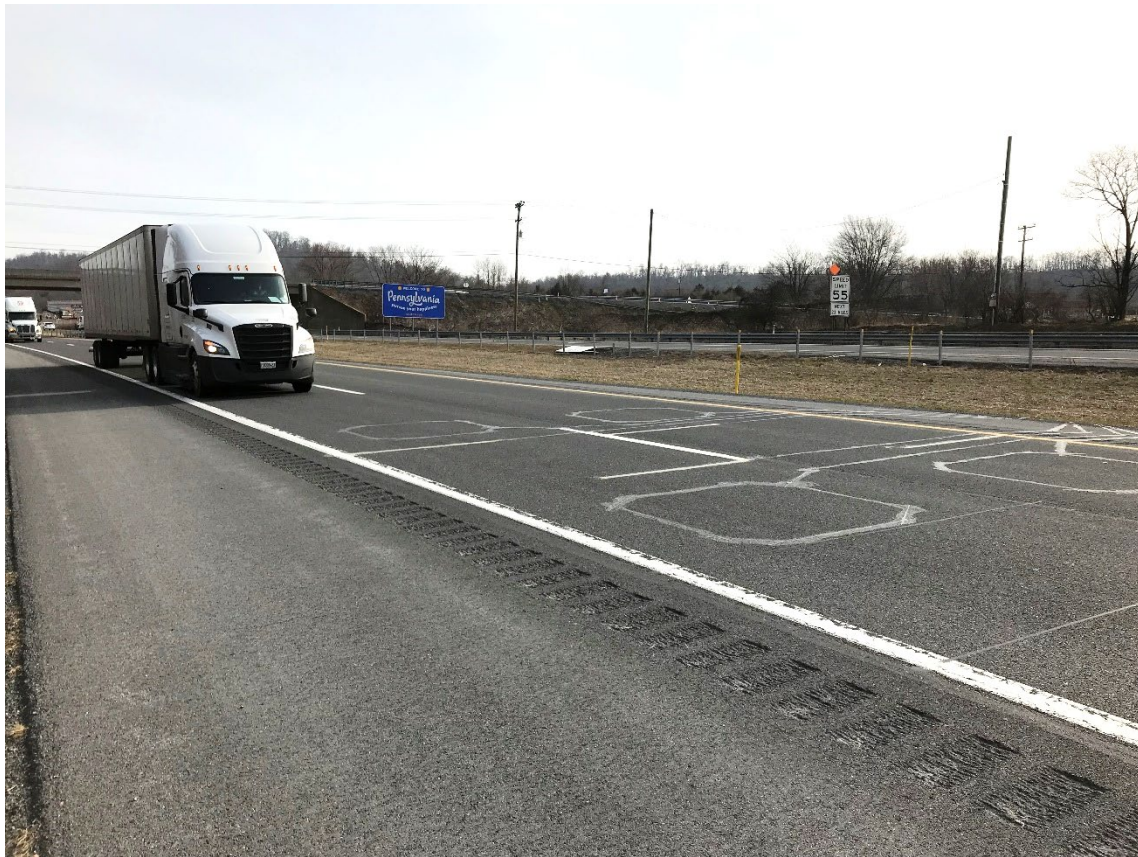
WIM 704 Sensor Arrays on I 70 in Fulton County
