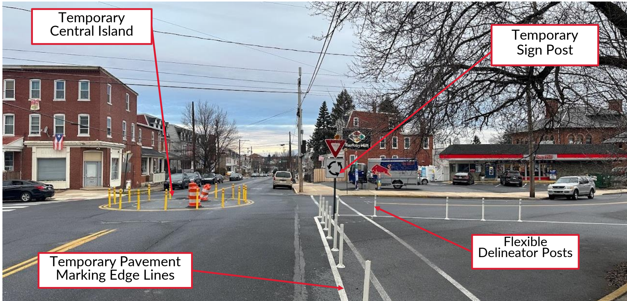
Elements of the temporary mini-roundabout installed in 2019
