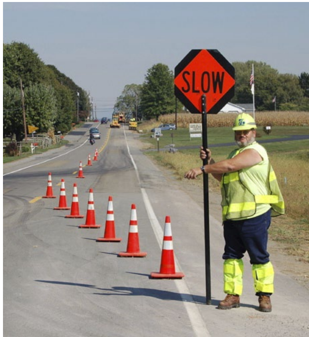
PennDOT's Flagging Handbook includes information for flaggers about basic positioning, proper attire, and the correct use of a STOP/SLOW paddle.
