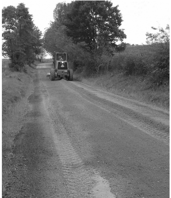
Excessive moisture during the "mud season" of spring creates ideal conditions for grading dirt and gravel roads.
