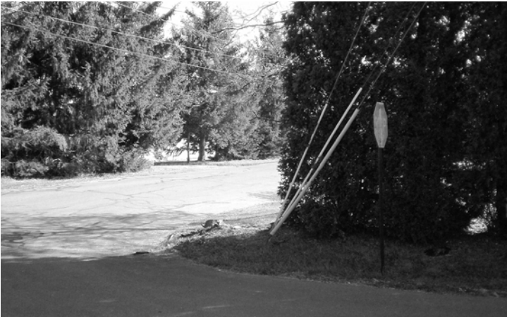
One tree had been removed, and a second was later removed to further improve sight distance – Clarion Borough, Clarion County
