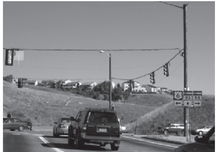
Traffic Signal Support – Strain Pole
