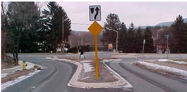
The curbing around the right-in/right-out island limits turning movements and may deter cut-through traffic.
