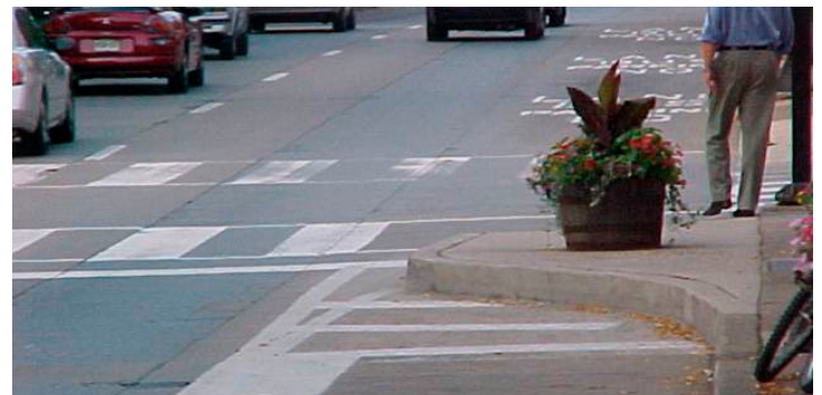
Bulb-outs, such as this one in State College, have proven to reduce the speed of traffic and improve pedestrian safety.
