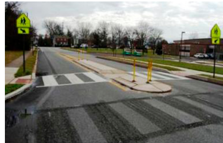
A crosswalk in Hatfield Township is shown before any traffic calming treatment (left) and after a pedestrian refuge median has been installed (right).
