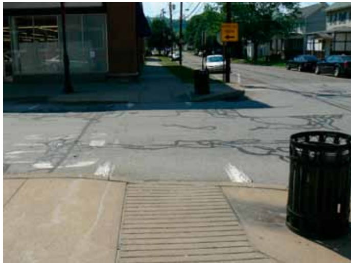
Example of a best-fit ramp installed in the 1990s.
