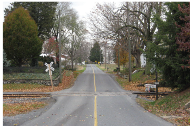
Single-line centerlines are prohibited, and railroad crossings with no signals or gates require the use of stop or yield signs.
