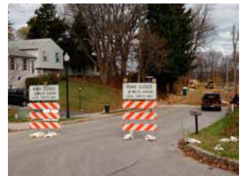
R11-3A road closed signs mounted on Type III barricades.
