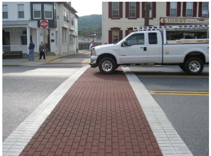
Example from Emmaus, Pa. This style meets current standards, as long as the transverse white lines are reflective.
