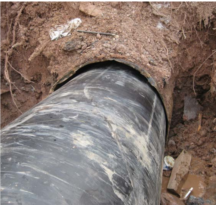
The HDPE lining is inserted snugly inside the metal pipe . . .
