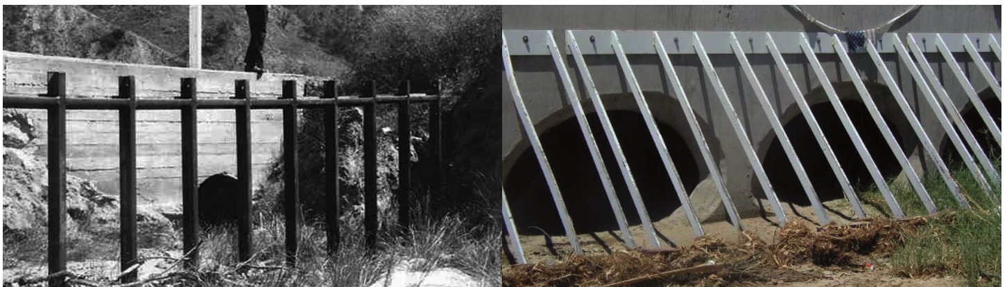
Figure 2 Debris racks (FHWA)
