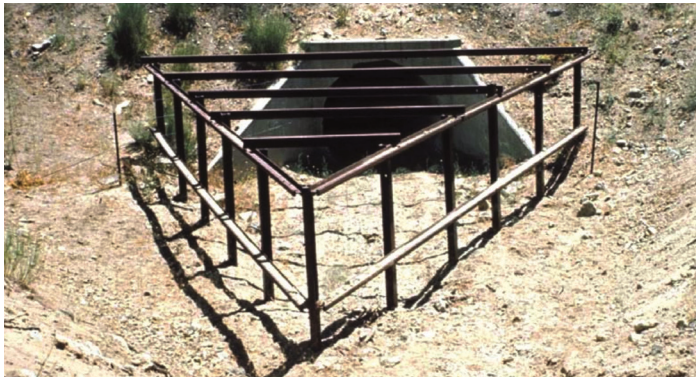
Figure 1 Upstream view of a steel debris deflector (FHWA)
