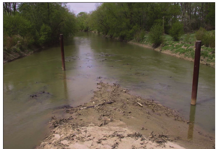
Figure 5 Debris deflectors for a bridge
