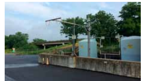
Through use of a spray bar, salt can be wetted after a load is on a truck.
