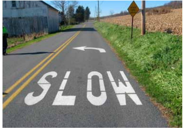
The SLOW curve pavement marking is an example of a roadway safety improvement.
