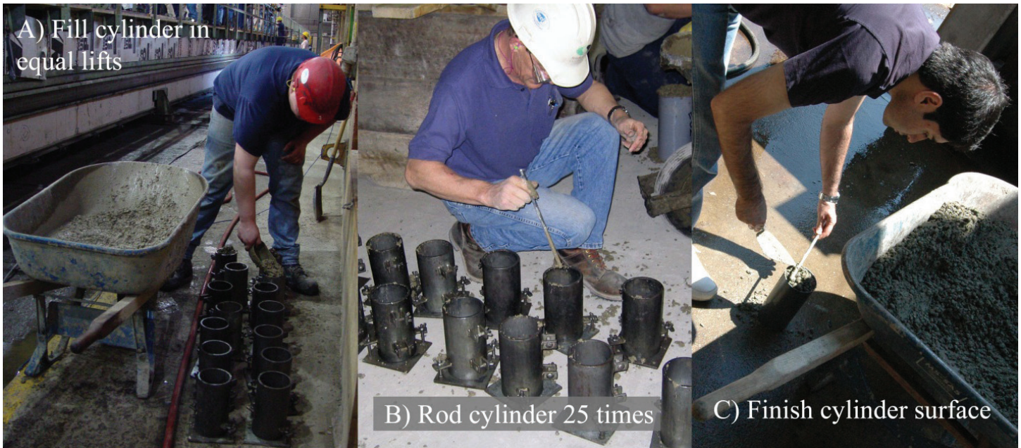
The concrete cylinders used to test concrete strength are fabricated on a site.
