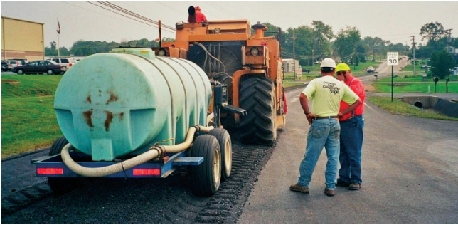
A nurse trailer containing calcium chloride is pulled behind a reclaimer on a pulverization FDR project in York County. The use of calcium chloride helped to provide dust control between the time the FDR was completed and a week later when the hot-mix asphalt paving on this industrial road was started. The calcium chloride stabilized base must cure for at least five days after final compaction.
