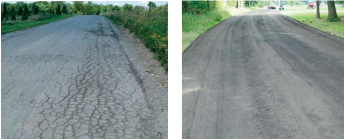
Schoonover Road in Graham Township, Clearfield County, before and after its calcium chloride stabilization FDR project.
